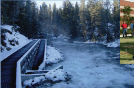
Fish ladder at low-head hydropower facility Fall River Rural Electric Cooperative, Idaho
